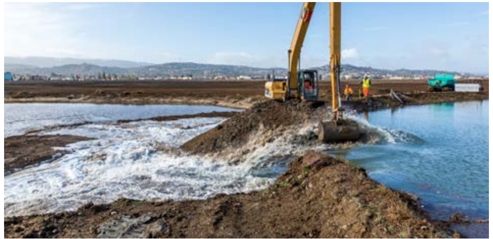
A levee breach at the Dec. 10 event caps a multi-year restoration that will return the diked-off site to tidal wetlands. Photo: Julie Kitzenberger
