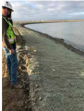
Internal levee rehabilitation in Alviso (USFWS)
