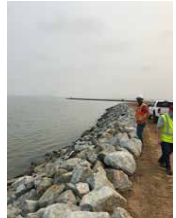
New levee armoring along the Bay in Menlo Park (USFWS)
